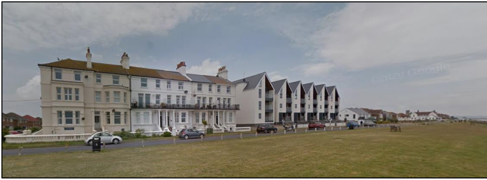
Fig.2 Four-storey developments to the south, facing towards Sandbanks
